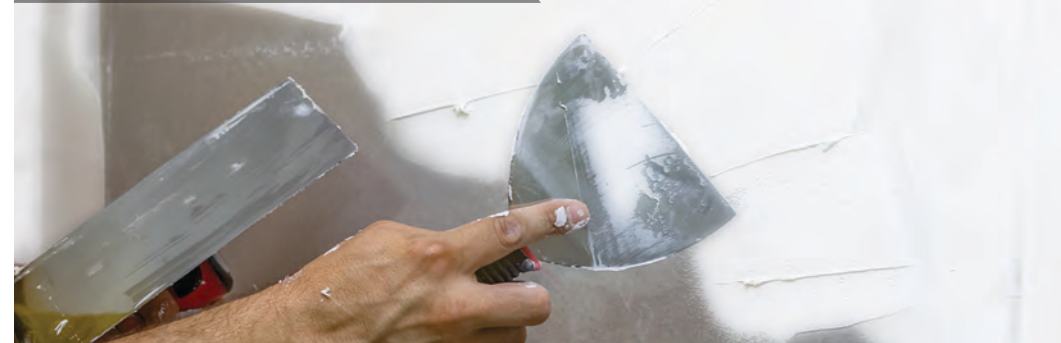
Closing pores using Wall Putty mix
